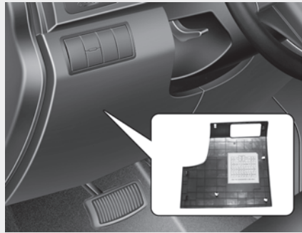
Inner fuse panel
